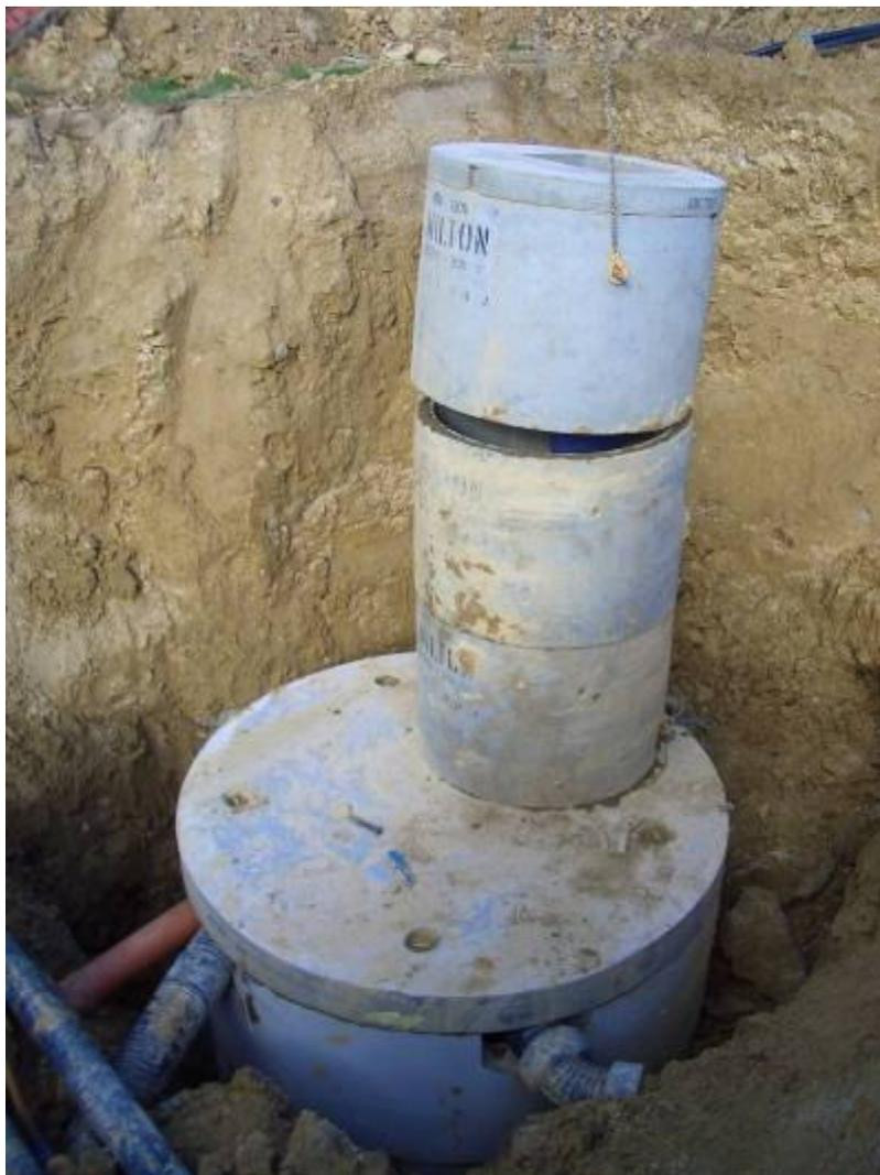
Collecting chamber being assembled for 'harvested' water to be pumped to a reservoir
